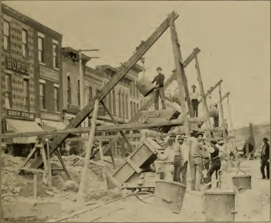
SEWER MACHINE AT WORK—AURORA, ILLINOIS.
